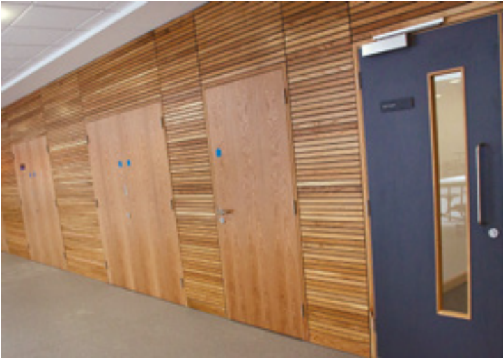
Store room doors using both lever handles and cylinder pulls. Where store rooms will be opened infrequently, cylinder pulls may be more appropriate and cost effective. In this specific example, the hardware chosen adds to the clean, flush, architrave free style of the project.
