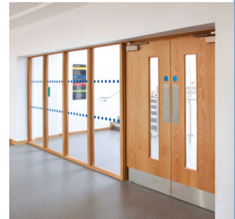
American white oak in a new academy in West Sussex. Where possible these doors are fitted alongside screens to allow for increased transition of light. These fire rated screens also create a feeling of openness and brightness conducive to a pleasant learning environment.
