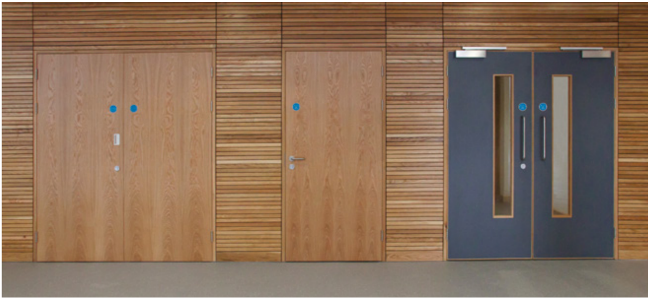
A combination of Formica Storm Grey laminate and American white oak veneered doors. Storm Grey laminate is complemented with exposed oak lippings, frames, architraves and glazing bead for circulation doors. Whilst contrasting crown cut, American white oak service and store room doors act as a way finding feature for students and teachers.
